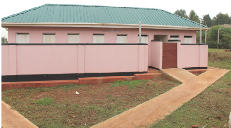
A new privacy wall around toilet block.
