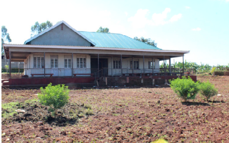
The clinic building seeing a lot of progress.
