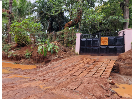
Please pray for a speedy job on our street repairs!!
