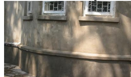
Restoration of front wall
