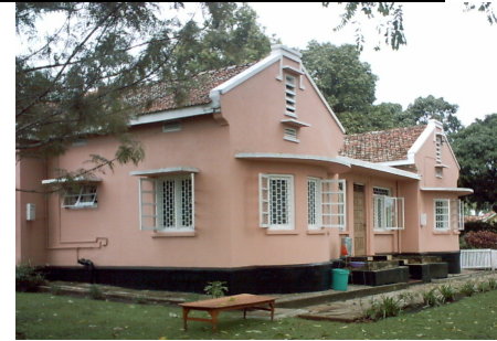
The front corner that had the big crack
