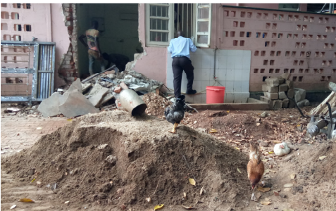
New Laundry floor prepped via outside wall
