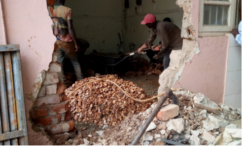
New laundry floor prepped via outside wall.
