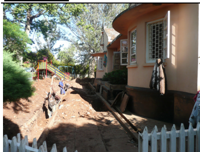
The trench being dug at the front.
