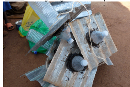
Above & Below: Bottle lights (water filled) installed in a village for the villagers to copy.
