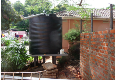
New tank and school room
