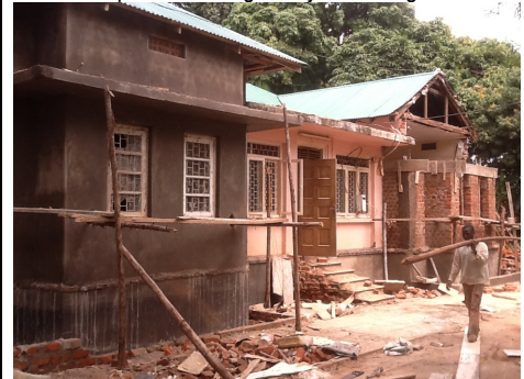
Above: House repairs - making good progress!!
