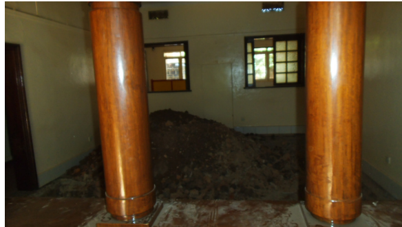
Above: Looking into the dining room from the front entry.
